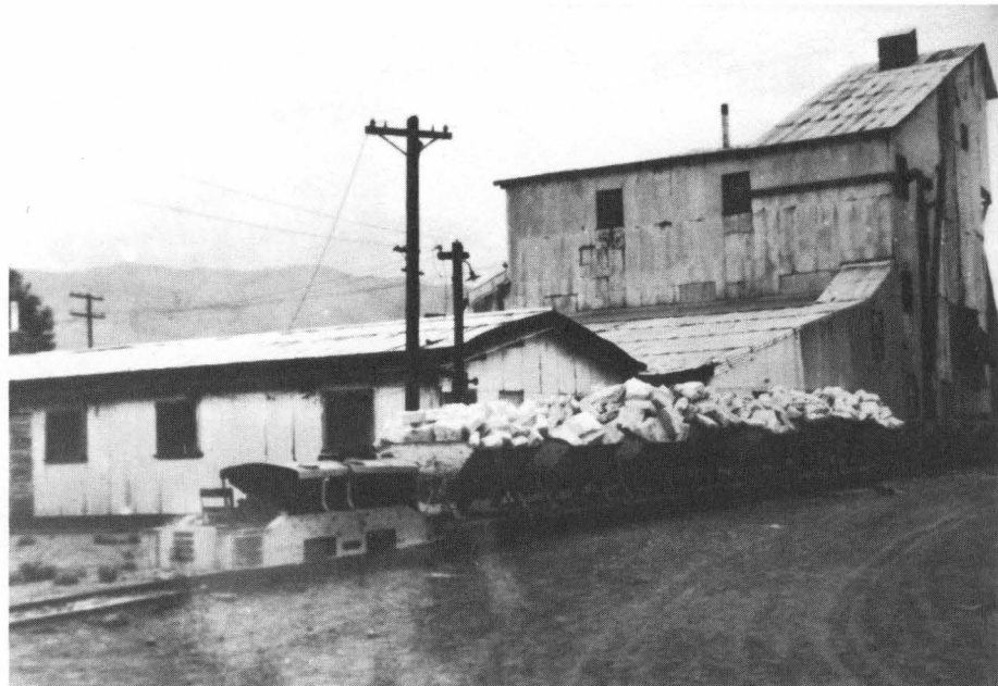
Fig. 1. Mill at Saltdale, February 1955. William Ver Planck, Calif. Division of Mines, courtesy Larry Bredenburg.
