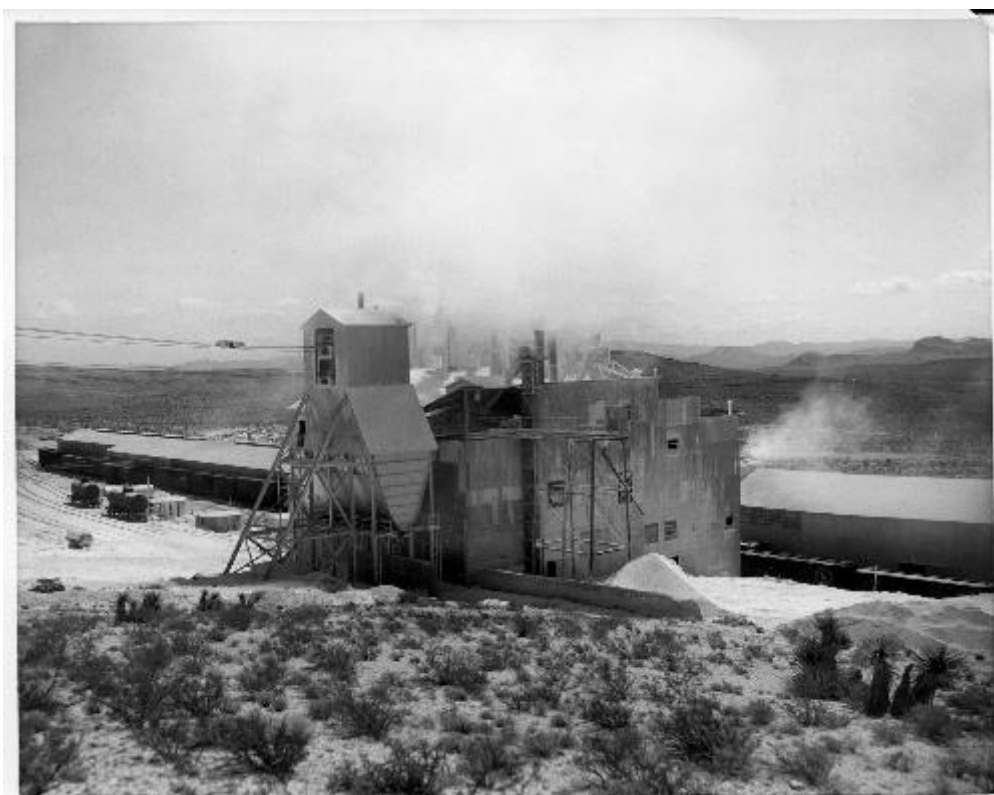
Figure 5. Blue Diamond Mill and Ore Loading Facility, from https://www.reviewjournal.com/uncategorized/southwest-of-las-vegas-village-of-blue-diamond-upholds-nevadas-legacy/ accessed Nov. 11, 2023. Open source for educational purposes, no copyright.
